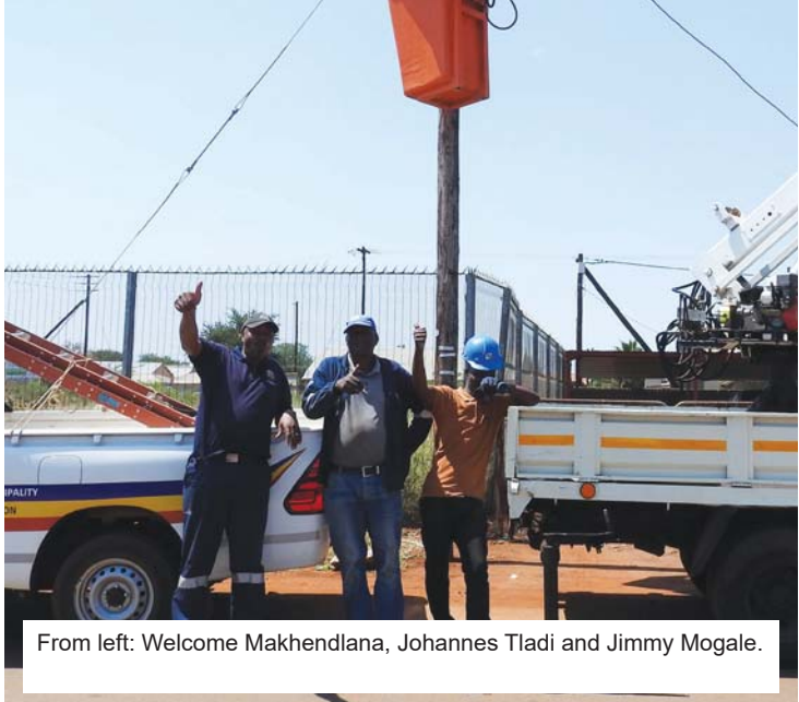
TLM assistant electrician Frank Monyeki busy changing the globes on the streetlights.
